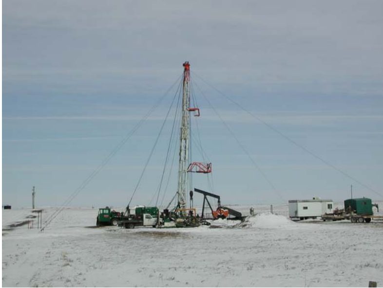
Figure 1. Workover of the CO2 Project #12 well in late February-early March 2003.
