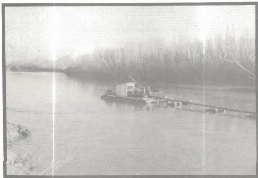
Figure 17. Sand pumping operation in the Blue River.
